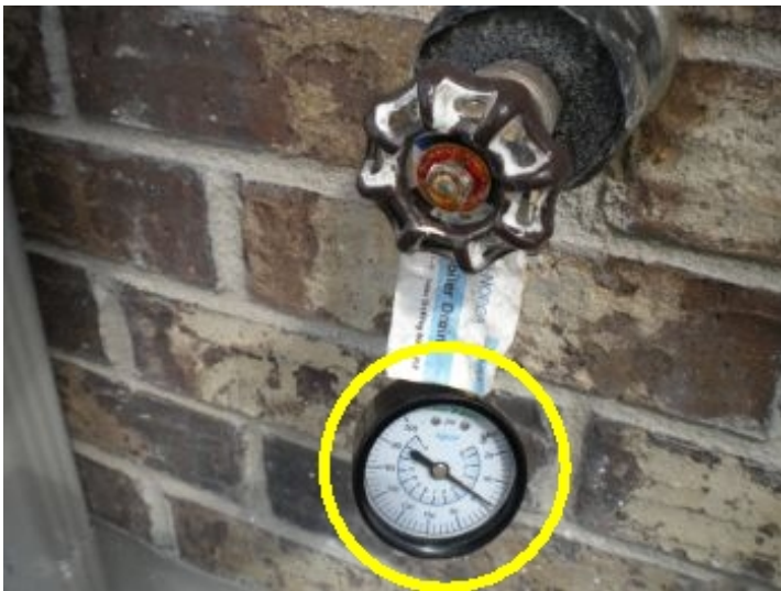
The anti static water pressure readings are typically at {40-80 psi} in the normal operating range. Water pressure registered 60 psi at time of inspection.
