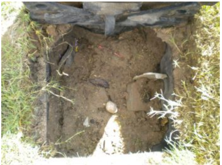
Was unable to inspect water meter due to being covered with dirt - Recommend cleaning area around water meter
