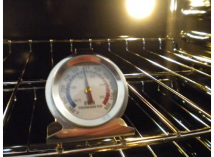
The oven was tested at 350 degrees for a {20} minute period and achieved a temperature of 340 degrees at time of this inspection. This is within the + or - 25 degrees standard.
