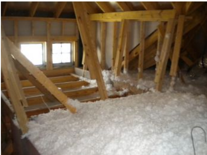
Unable to determine condition of anything under blown-in insulation.
