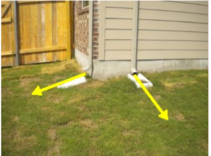
Gutters missing one or more downspout extensions - Recommend installing 6 ft downspout extensions to move water a way from foundation
