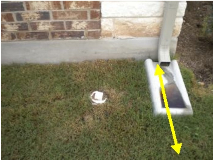
Gutters missing one or more downspout extensions - Recommend installing 6 ft downspout extensions to move water a way from foundation
